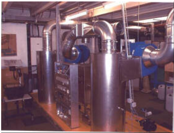
Figure 6. Thermal Diode Wall System
