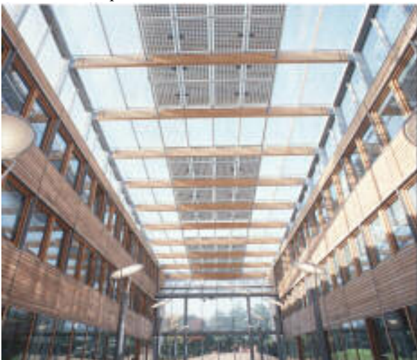
Figure 1. Entrance Hall at the Jubilee Campus Showing Ceiling PV Panels
