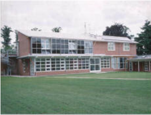
Figure 2. Marmont Centre for Renewable Energy Showing Wall PV Panels
