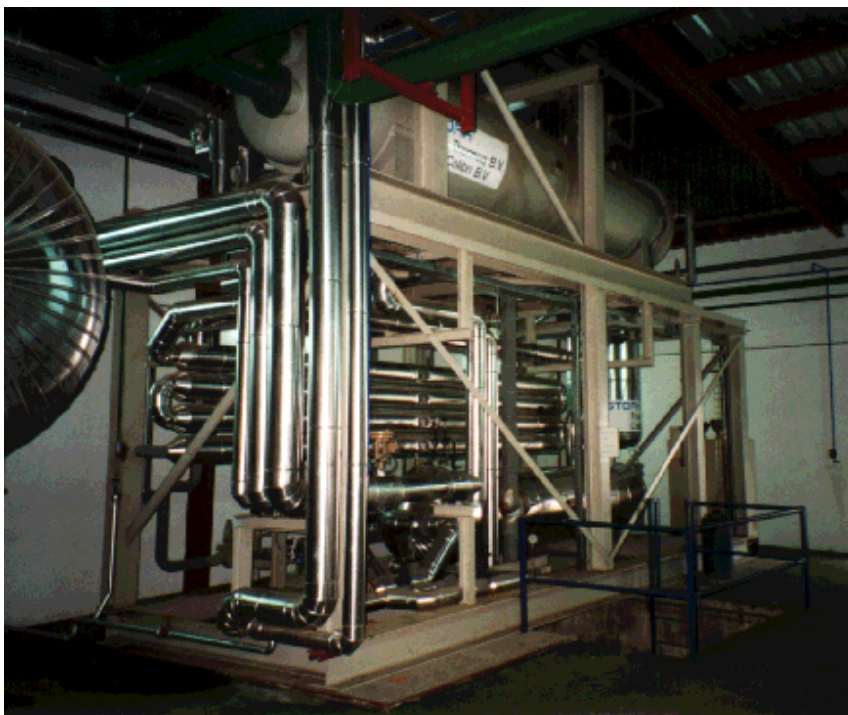
Figure 5 The ARP installed in a vegetable freezing factory in Talavera (Spain)
